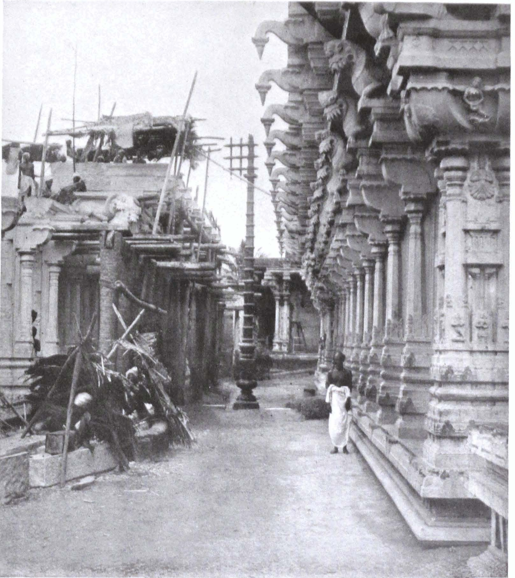
MODERN HINDU TEMPLE AND ITS BUILDERS (KALIARKOVIL, MADRAS).
